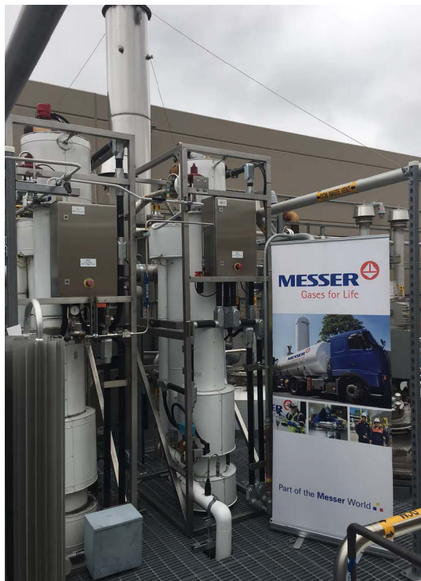
Bachem installed two cryogenic condensation vapor emission control modules at its facility to remove more than 99.8 percent of VOCs from its process stream. One unit operates at a time. The second unit is on standby and takes over when the first goes into defrost mode.
